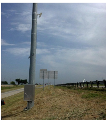
Figure 3-7. Bluetooth Detection Technology is a Low-cost Method of Collecting Anonymous Point-to-Point Travel Time Data
